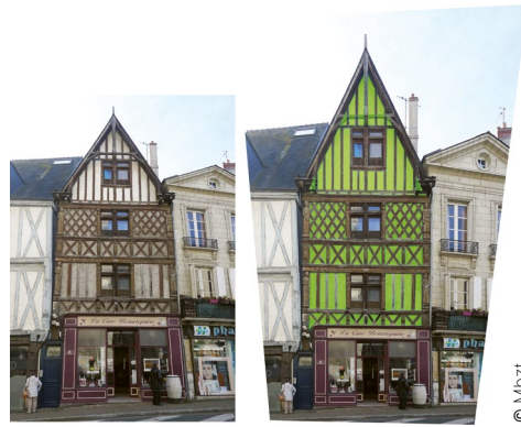
Upper left: original photograph. Upper right: facade transformed into a front view with survey of the rendering (green surface)
