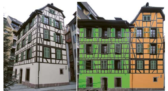
Above, on the left: original photo. On the right: straightened photo with structure of the building and survey of the plaster surfaces (in green and orange).
